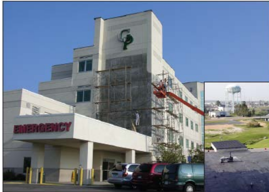
Hurricane Katrina – 2005 Garden Park Medical Center Cladding & 6" of Flooding
